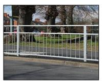
Pedestrian guardrails are designed to protect adults and children at road junctions and crossing points, whilst allowing good visibility from a motorists view point.
