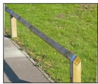
Trip rail fencing, also known as knee rail fencing, is commonly used to mark the boundary in places such as car parks and alongside pathways. It is also used to prevent cars from parking on grass verges.
