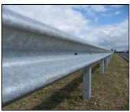
Vehicle Restraint Systems (VRS) or Safety Fences are used mostly on motorways, dual-carriageways, junctions and approaches to roundabouts. Their main purpose is to restrain or redirect errant vehicles from crossing central reservations into the path of other vehicles or from leaving the road following accidents or collisions.
